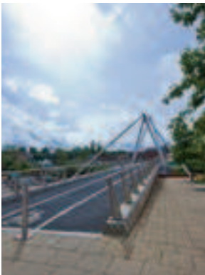
Landmark bridge structure
