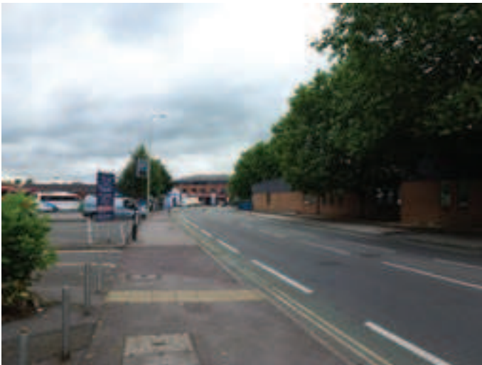
Opportunity to improve Oxpens Road public realm
